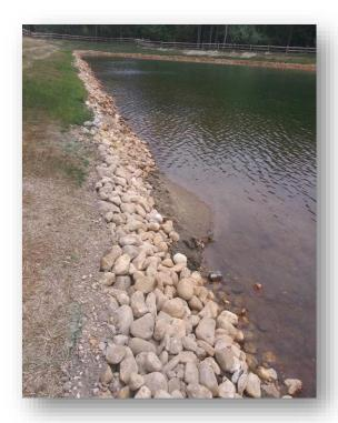
Retention ponds will act as a pollutant treatment basin as well as a collection location for heavier flows, reducing peak runoff rates downstream. Retention ponds, if not properly maintained, can increase pollutant discharge downstream, increase the instability of downstream channels, raise the risk of downstream flooding.
